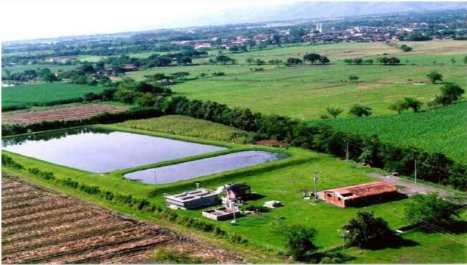
Figure 2. WSP system at Ginebra in southwest Colombia (population 9,000; wastewater flow 27 l/s) comprising an anaerobic pond and a facultative pond. The WSP effluent is used for the irrigation of sugar cane.
